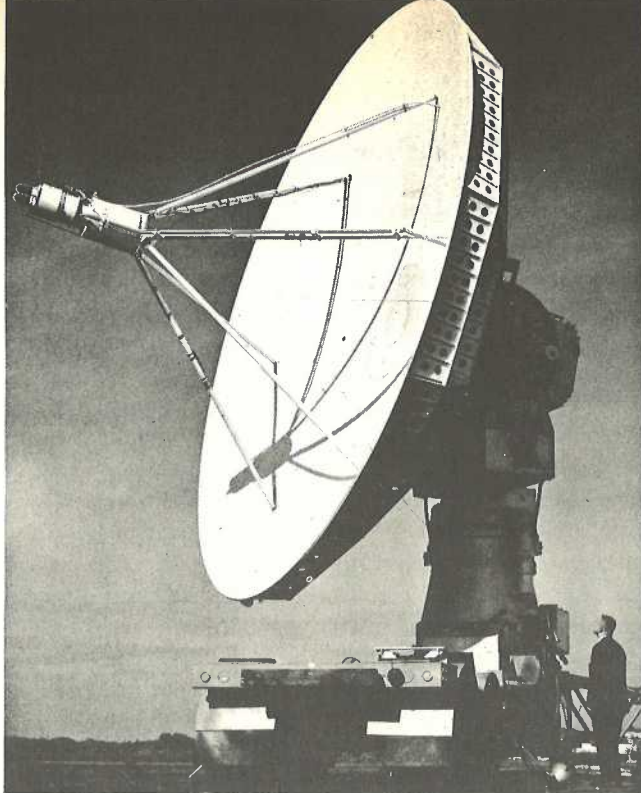
Syncom's transportabele antenne te New Jersey. diameter 10-m
